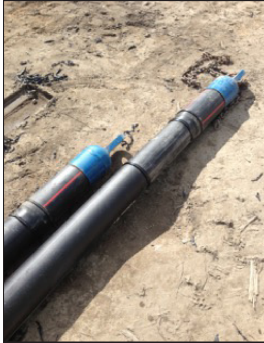
HORIZONTAL DIRECTIONAL DRILLING 4 X 6 POLY-FLO® PIPE PULLING HEADS
