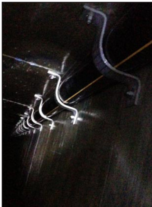
HORIZONTAL PIPE SUPPORTS
