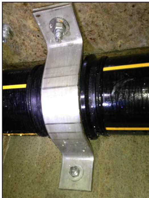
RESTRAINT FITTING
